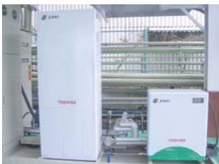
LPG-reforming type stationary fuel cell system
