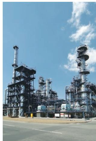
Because making low-benzene gasoline and sulfur-free gasoline requires refineries to use more energy compared to conventional gasoline refining, we try to make up for this by saving energy through methods such as waste heat collection, heat collection using heat exchangers and reduction of steam loss.
