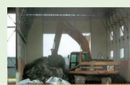
Mixing the soil with calcium oxide
