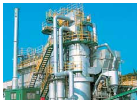
NIPPO Corporation's Soil Remediation Center equipped with this thermal soil-drying plant
