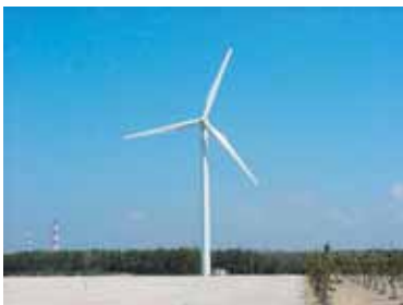
The wind power generation unit at the Akita Oil Depot
