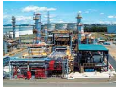
A ROK-Finer® facility at the Sendai Refinery
