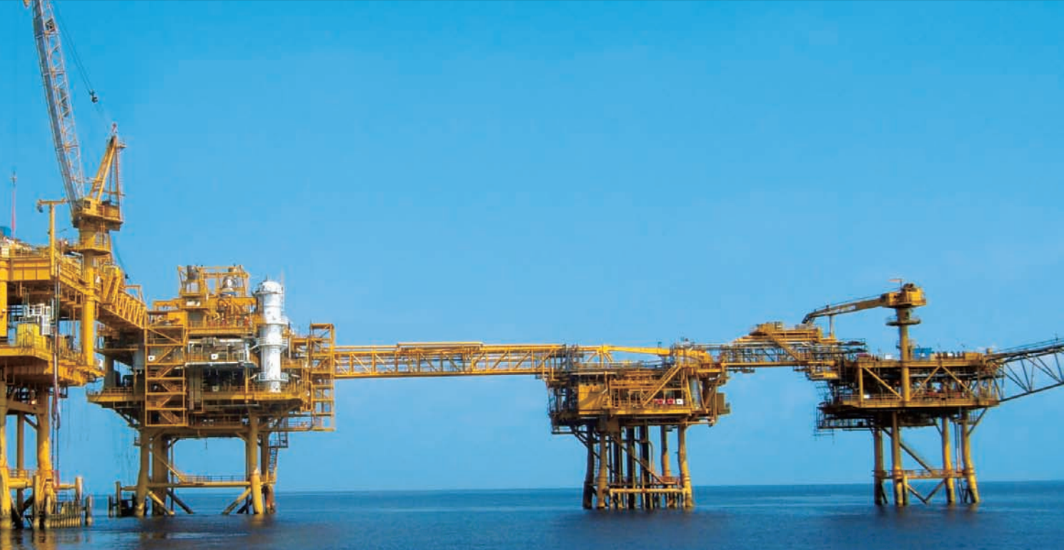
Drilling platform in Vietnam's Rang Dong oil field
