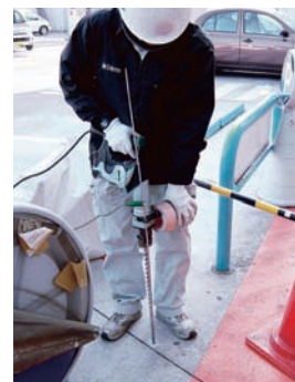
Gas density inspection underway at an operating service station
