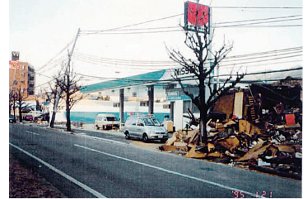
A service station after being verified as safe following the Great Hanshin Awaji Earthquake in January 1995 (Photo provided by Tatsuno Corporation)
