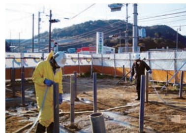
Soil remediation underway at an idle service station site
