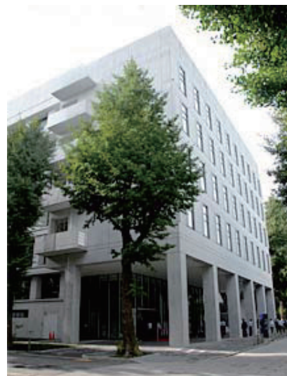
The Environmental Energy Research Building was newly constructed in fiscal 2011 to house the ENEOS Lab
