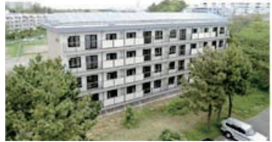
Verification testing on a SOENE plus renovation project at our Shiomidai company-owned apartments
