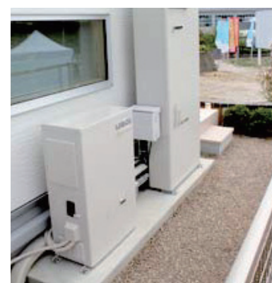
An ENE-FARM residential use fuel cell system
