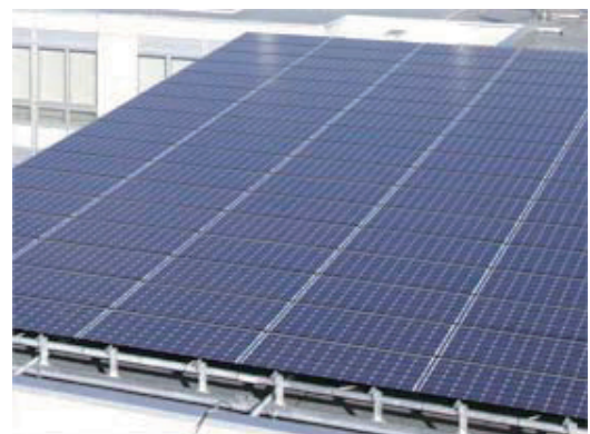
A photovoltaic power generation system installed atop an apartment building
