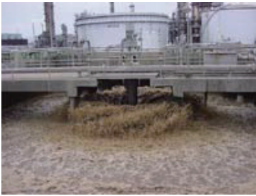
*1: Activated sludge treatment unit
