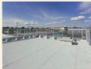
Rooftop space for temporary evacuation during a flood
