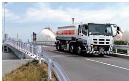
A bridge constructed between the west and east sides of the refinery to ensure tank trucks enter and exit the refinery without passing through the nearby residential area
