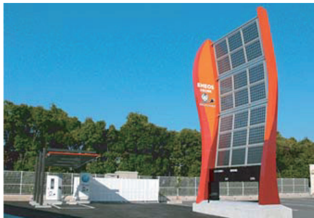
The solar panels and rapid recharging equipment for DD Energy Mall Yahata-Higashida Service Station
