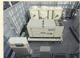
Water tank, generator and ENE-FARM
