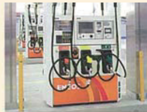
Watertight fuel dispensing equipment
