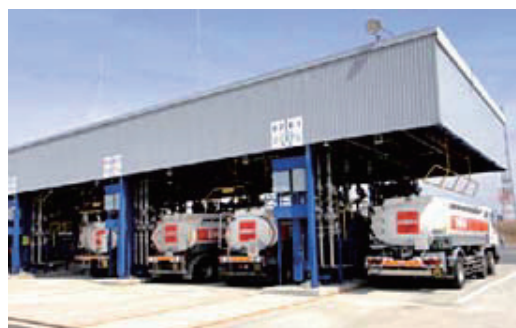
The temporary loading facility completed in just two weeks
