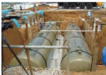
Tank replacement work in progress
