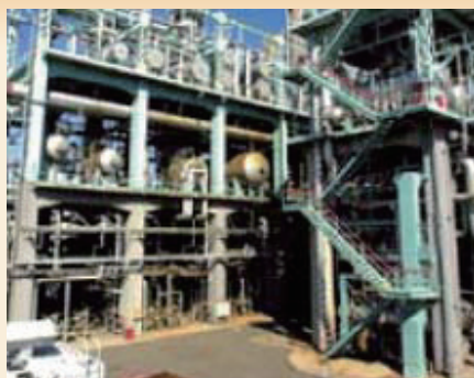
Ethylene manufacturing equipment at the Kawasaki Plant
