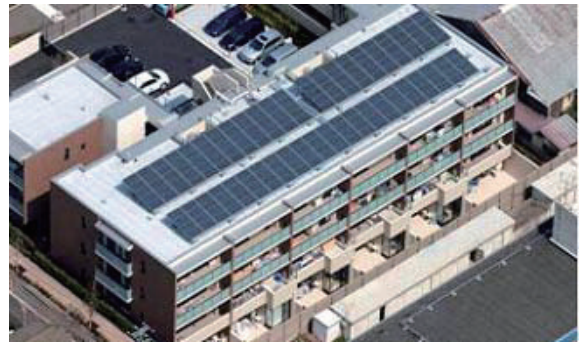
Condominium building example Condominium building in Tokyo Operator: The Sankei Building Co., Ltd. 1.29kW per unit (215W x 6 modules) x 33 units Total: 42.57kW
