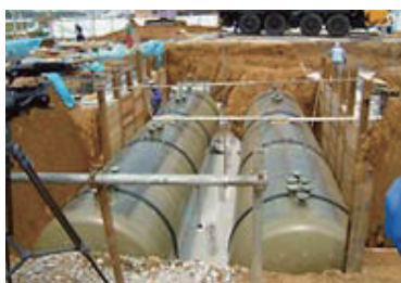
Tank replacement work in progress
