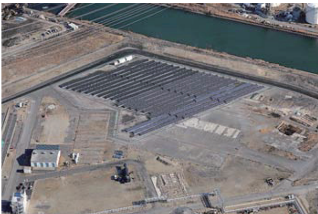
Sendai Mega Solar Power Plant
