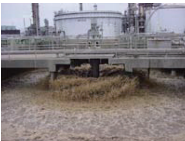
*1: Activated sludge treatment unit
