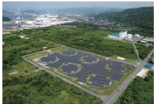
Kudamatsu Mega Solar Power Plant
