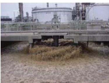
*1: Activated sludge treatment unit
