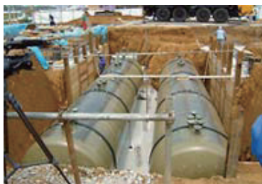
Tank replacement work in progress
