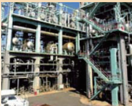
Ethylene manufacturing equipment at the Kawasaki Plant
