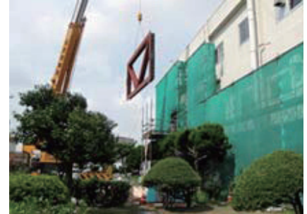
Seismic reinforcement of buildings
