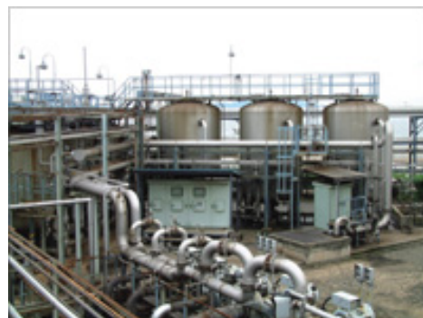
2: Activated carbon adsorption unit
