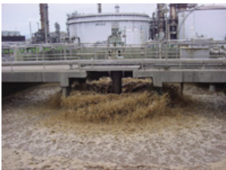
*1: Activated sludge treatment unit
