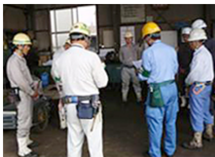
Safety check before work
