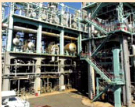
Ethylene manufacturing equipment at the Kawasaki Plant
