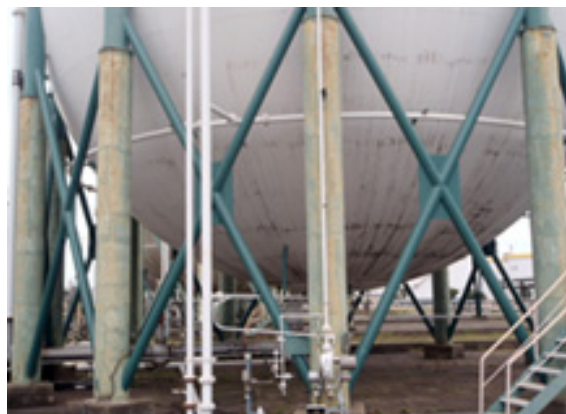
Example of brace retrofitting for a spherical tank
