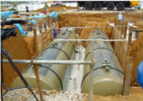
Tank replacement work in progress
