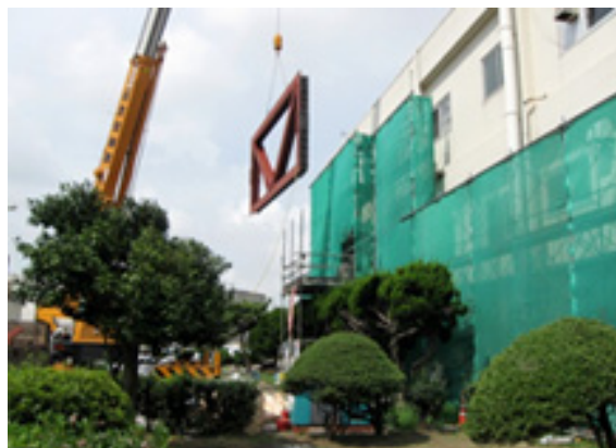
Seismic reinforcement of buildings Example
