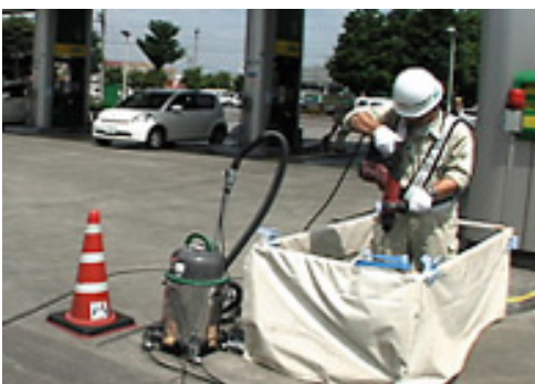
Soil survey work in progress
