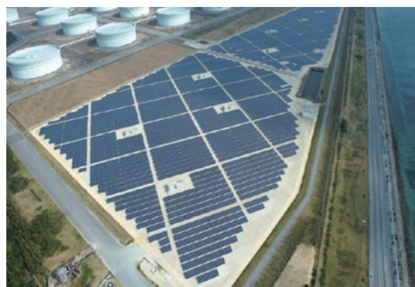
The Uruma Mega Solar Power Plant is the largest in Okinawa Prefecture, generating 14.60 million kWh of electricity per year, or enough to power 4,000 homes over the same period.
