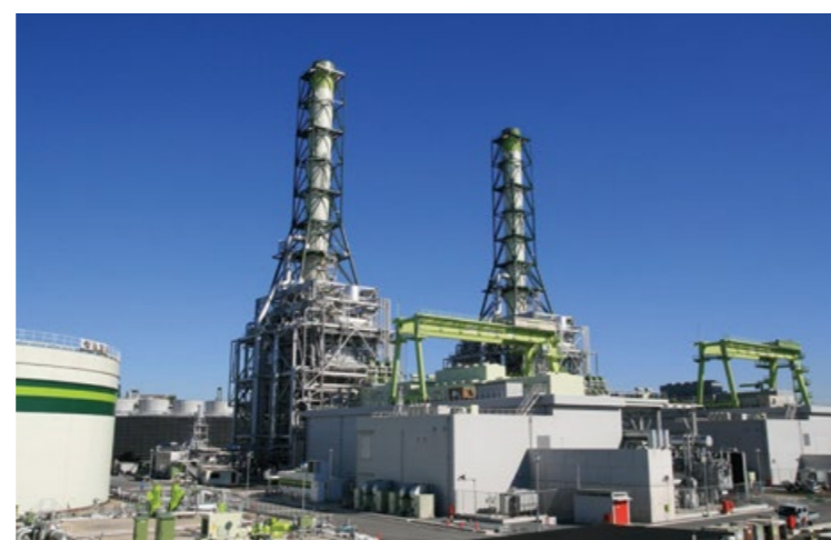
Kawasaki Natural Gas Power Plant
