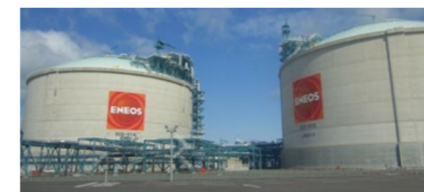
The Hachinohe LNG Satellite Terminal has a storage capacity of 280,000 kl of LNG.
