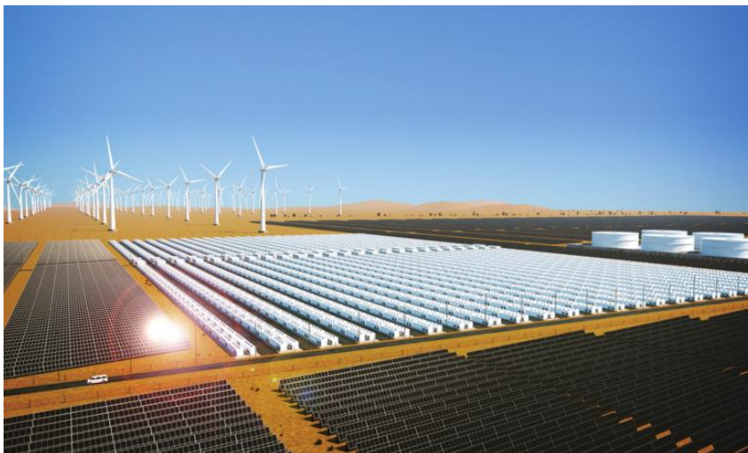
Image: Wind power 21km x 21km, solar power 7km x 7km, Direct MCH ® electrolyzer 700m x 400m, Toluene/MCH tank 300m x 400m
