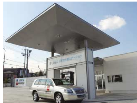
"JHFC Yokohama Asahi Hydrogen Station", which supplies hydrogen to fuel cell vehicles demonstrating their viability driven on public roads
