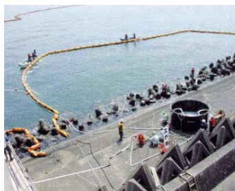
Practice drill for deploying an oil fence to prevent water pollution from oil spills
