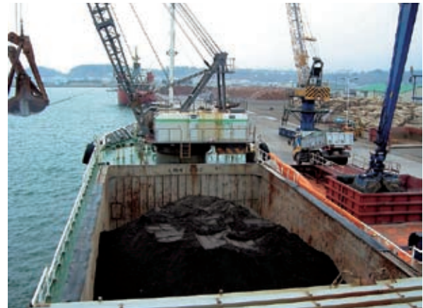
Loading intermediate treatment soil onto the ship (to deliver as raw material for cement)
