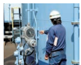
Inspector carries out a safety check
