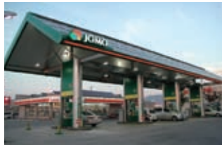
JOMO service station with solar panels
