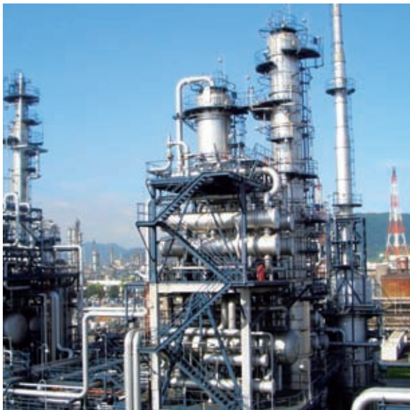
Sulfur-free gasoline production units
