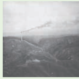
Giant smokestack at the Hitachi Mine
