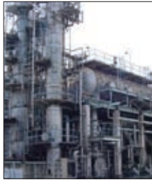
Sulfur recovery and flue-gas desulfurization equipment
