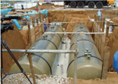
Tank replacement work in progress
