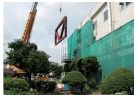
Seismic reinforcement of buildings Example
