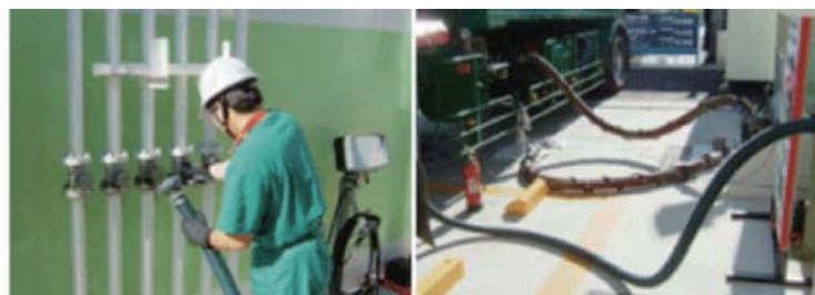
Capturing hydrocarbon vapors
