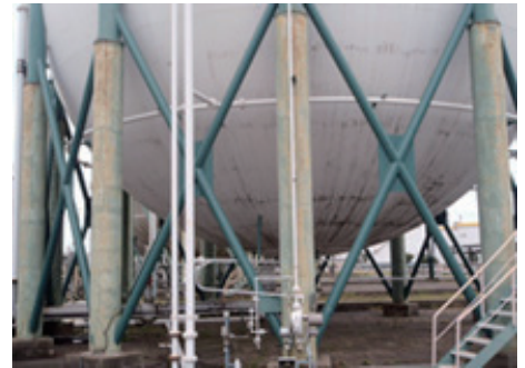
Example of brace retrofitting for a spherical tank
