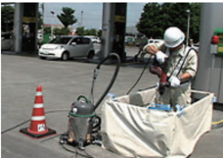
Soil survey work in progress
