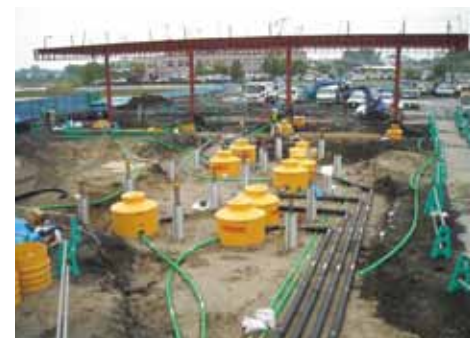
Installation of flexible resin pipes
