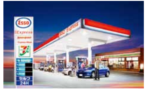
Express brand self-service station
